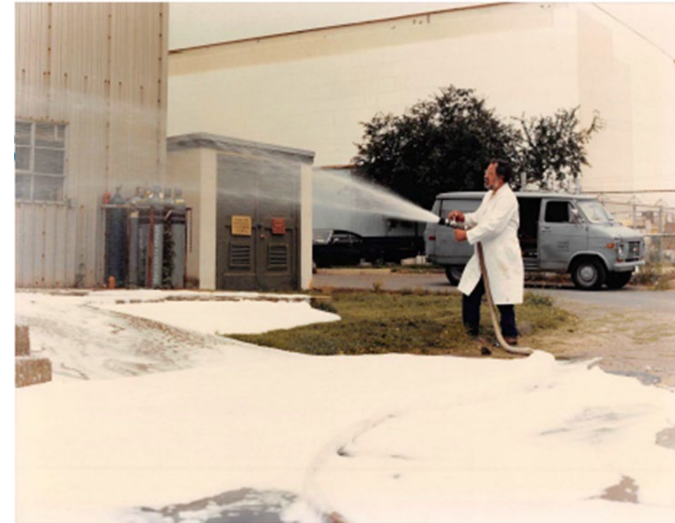
Early foam testing at Naval Research Laboratory – DC
